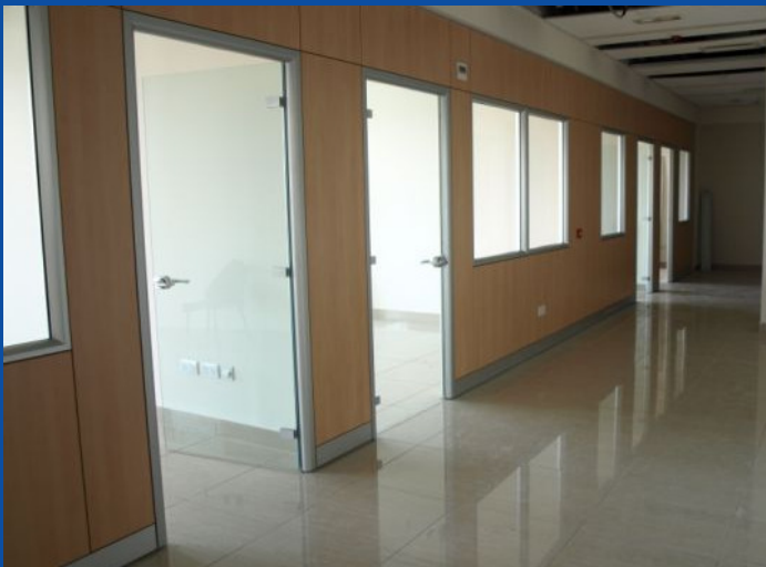
A first glimpse of the new EASO offices: works on the new EASO premises are nearing completion.
